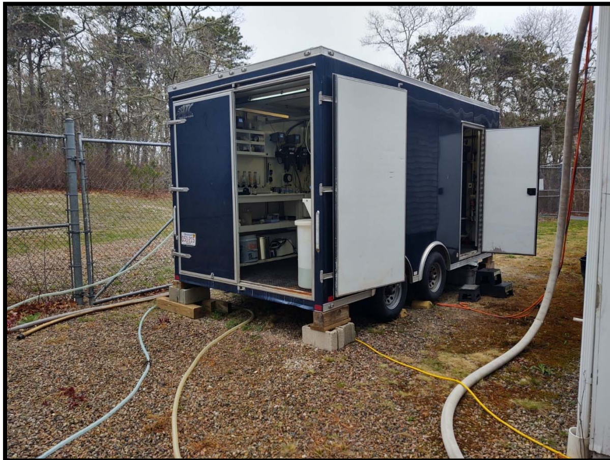
Figure 2.04: Greensand Pilot Trailer at Hyannisport Station
