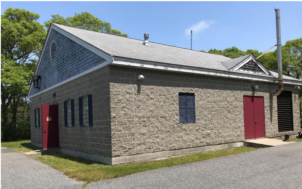
Figure 2-1: Existing Straightway Treatment Facility
