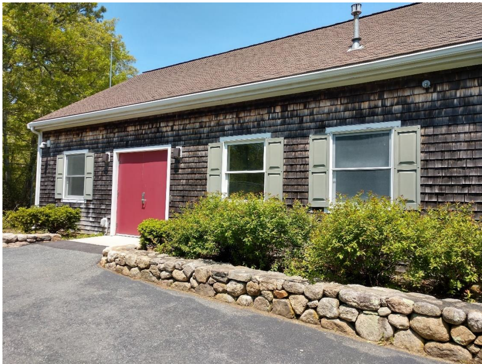
Figure 2-2: Existing Hyannisport Treatment Facility
