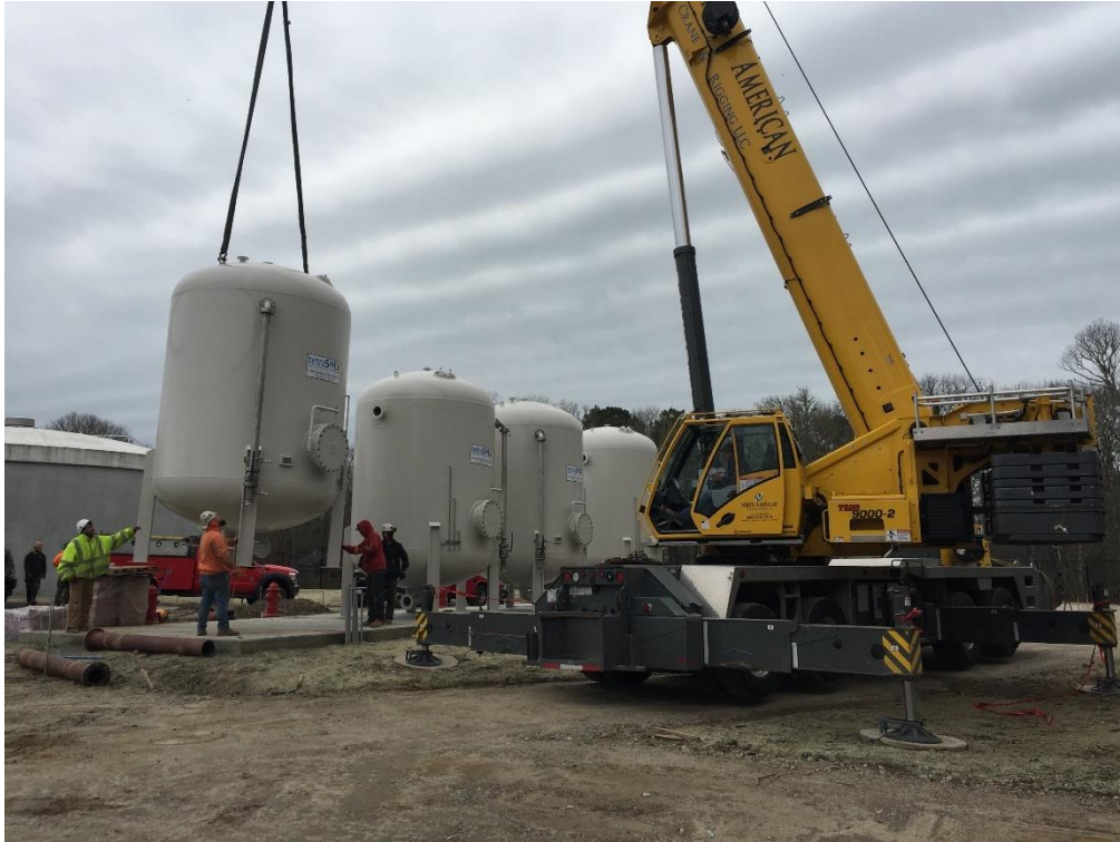
Figure 2-3: Installation of Seasonal Interim GAC Filters at Straightway
